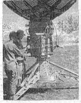
CHECKING THE WEATHER—Staff Sergeant Richard Roberts (Atkinson, Neb.), left, and Specialist 5 James Kelly (Klamath Falls, Ore.) of the meteorological section check out the Rawin Set (radio receiver) prior to sending a transmitter aloft to check weather conditions.
